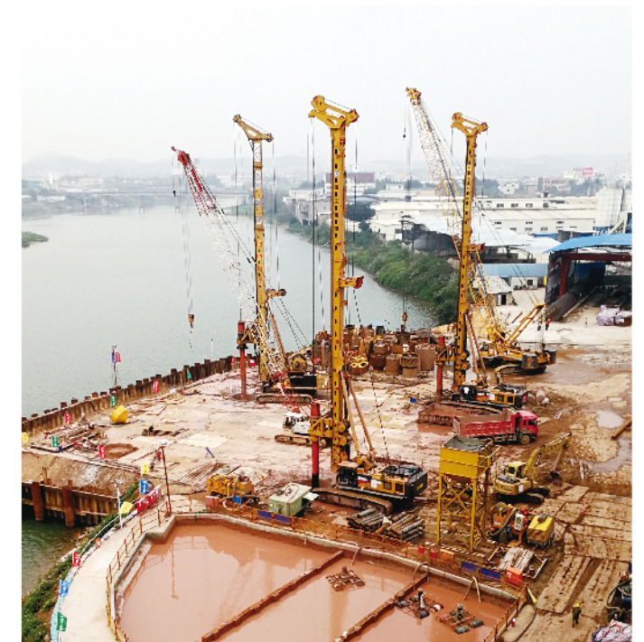
XR550在广东广州西江特大桥施工 XR550 work in the construction of Xijiang grand bridge in Guangzhou, Guangdong
