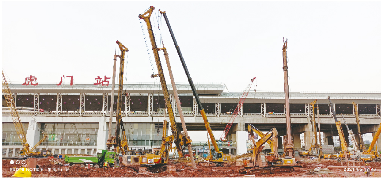
徐工旋挖钻机助力东莞虎门站施工 XCMG rotary drilling rigs help the construction of Humen station in Dongguan
